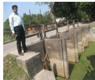
Photographs 3-5. Small and shallow sluice gates from Terokhada Upazila of Khulna District (Left and middle) and Tala upazila of Satkhira District (Right)
