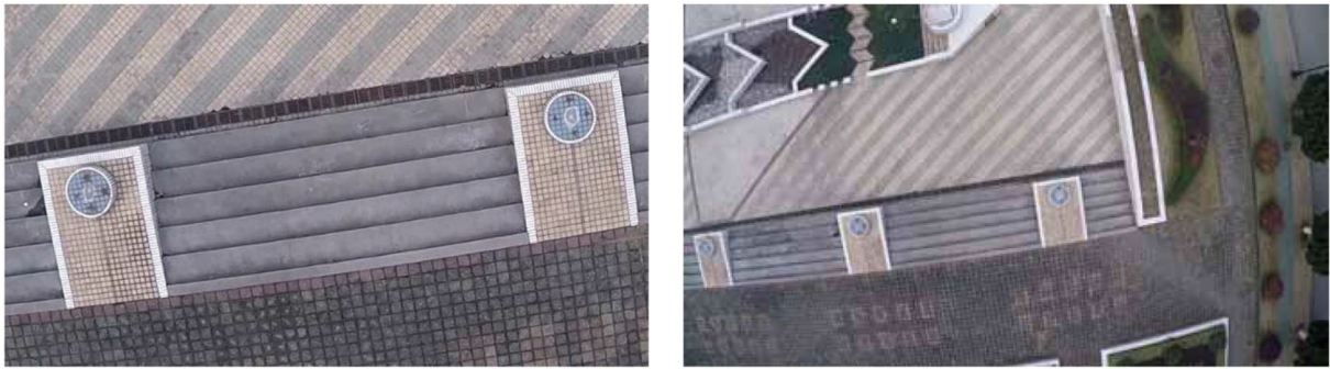
FIGURE 11 Images taken when the UAV panned and climbed.
