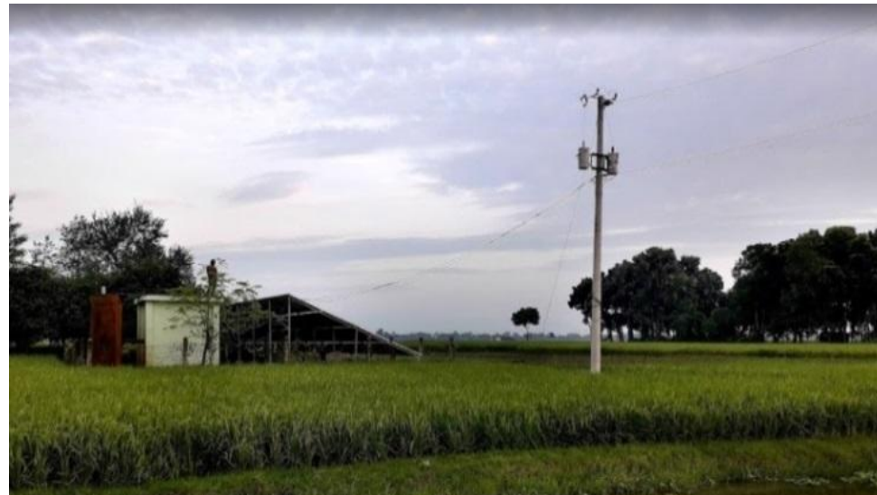
Fig. 5. First SIP grid integration piloting site in Bangladesh
