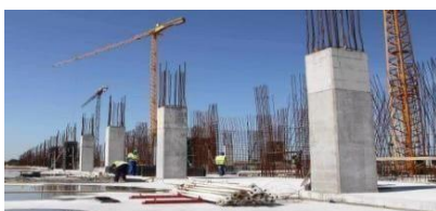
Fig. 3. Reinforced concrete column
