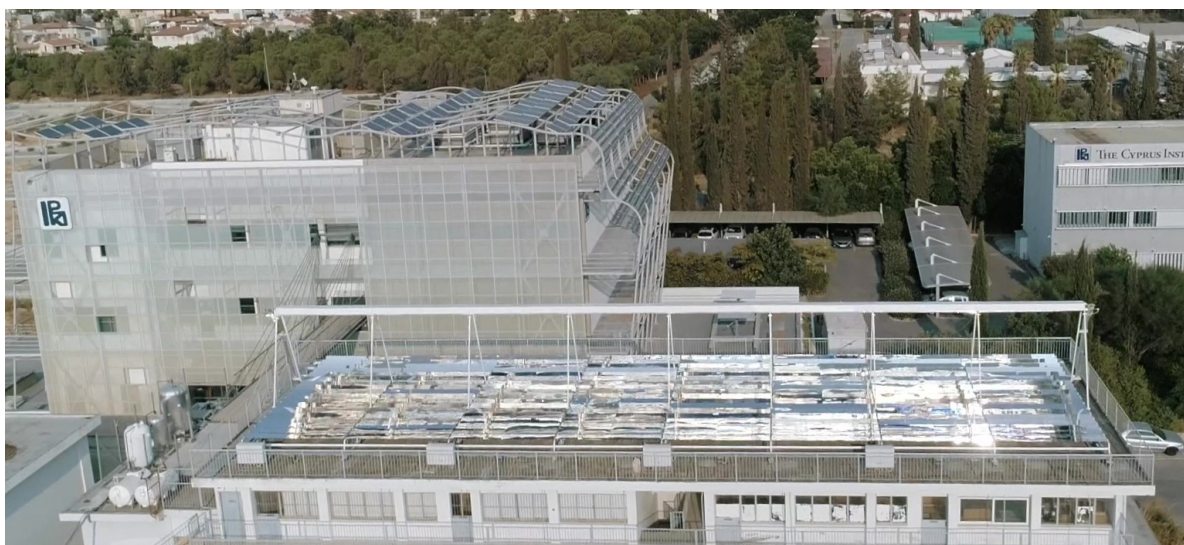
Figure 1. LFR collector at the Cyprus Institute and Novel Technologies Laboratory (NTL) building in the background on the left.
