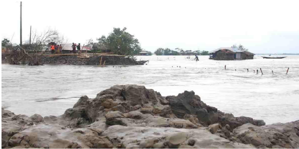
Photograph 2. Tidal surge during cyclone AMPHAN broke the embankment on Kholpetua River and flooded hundreds of houses in Napitkhali area of Gabura union in Shyamnagar upazila of Satkhira district. Photo Credit: UNB [41]
